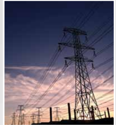
Electric utility substations Switchgear
