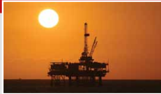
Oil and gas pipelines Offshore platforms
